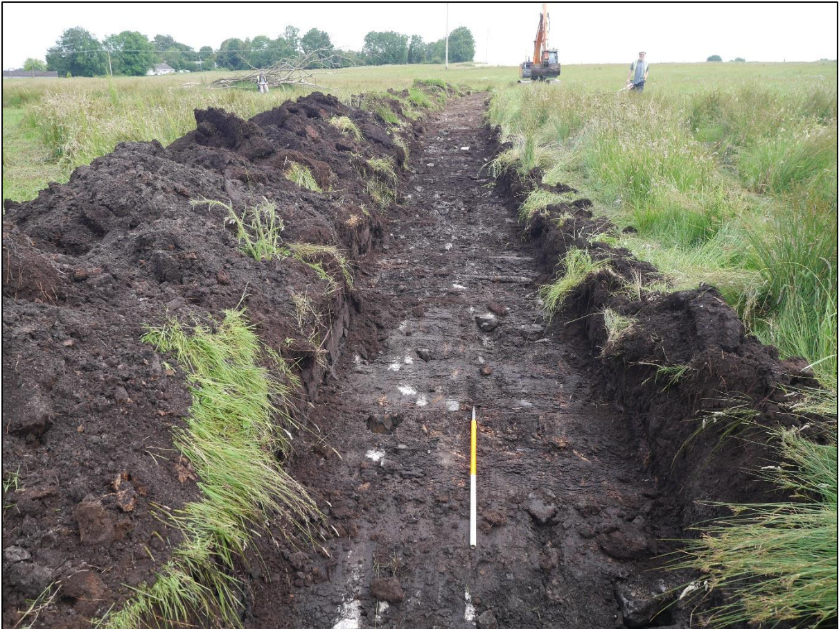
Plate 19: Ground conditions in the southern part of Cornacarta, this example from Trench 104, facing north.
